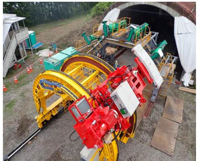
Photo 6. Erection machine for multi-divided precast lining
