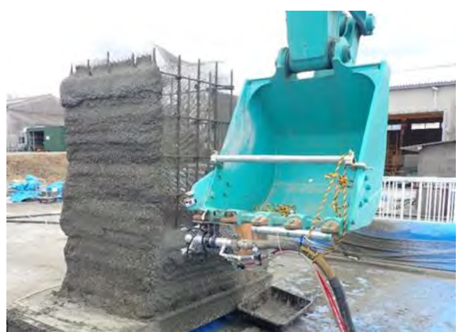
Photo 10. Direct print molding of buried formworks
