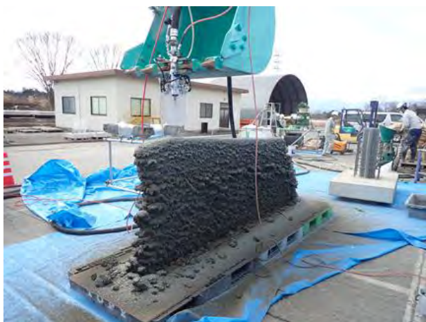
Photo 9. Direct print molding of a wall
